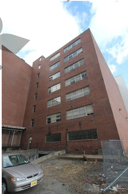
Photo 6 - West elevation, looking northeast.
