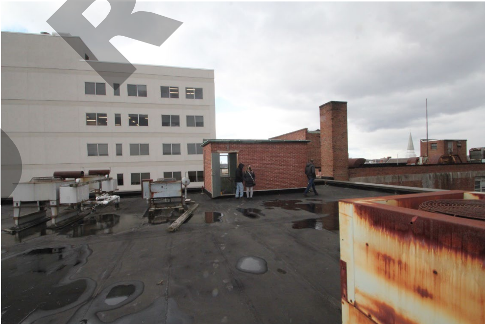
Photo 26 – Roof, looking west.
