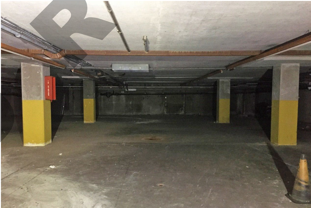
Photo 24 – Basement-level parking garage, looking north.
