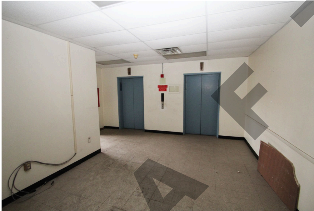
Photo 19 - 4 th floor, elevators, looking south.
