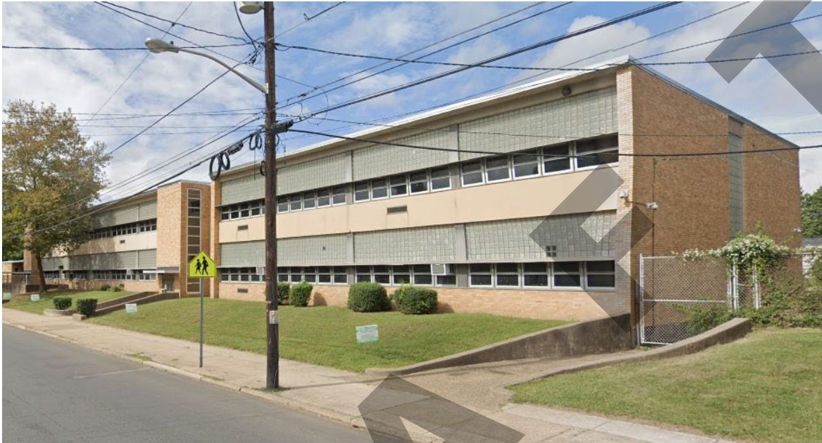
Figure 18 – Stokes Elementary School at 915 Parkside Avenue in Trenton, NJ, designed by Micklewright & Mountford and built 1950-53 (Google Street View).
