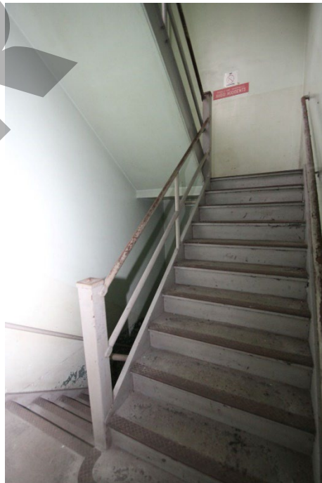
Photo 14 - 2 nd floor, stair, looking south.
