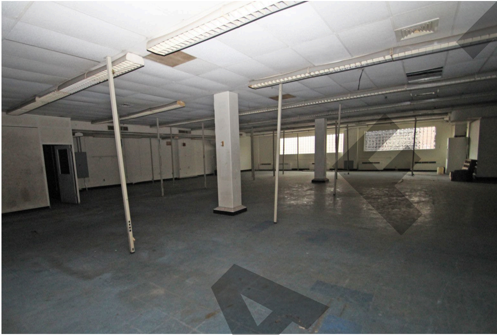
Photo 13 - 1 st floor, office area, looking southwest.
