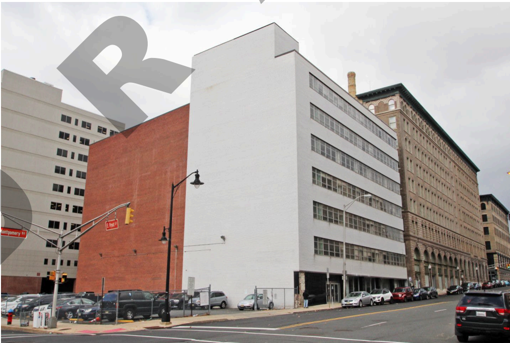
Photo 8 - South elevation, looking northwest.
