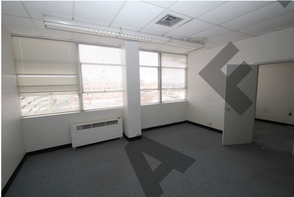
Photo 23 - 6 th floor, private office, looking southeast.
