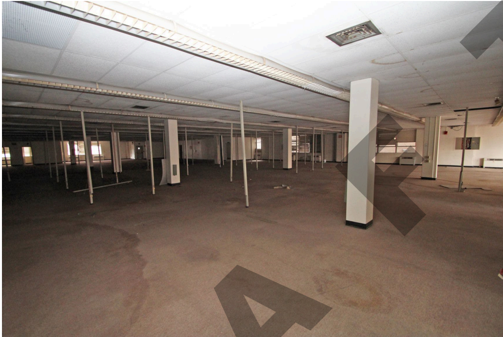
Photo 15 - 2 nd floor, office area, looking northwest.
