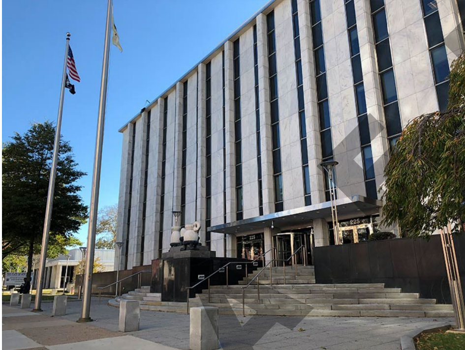
Figure 12 – Department of Education Building (now the Office of the Governor) at 225 W. State Street in Trenton ( njstatehousetours.org ).
