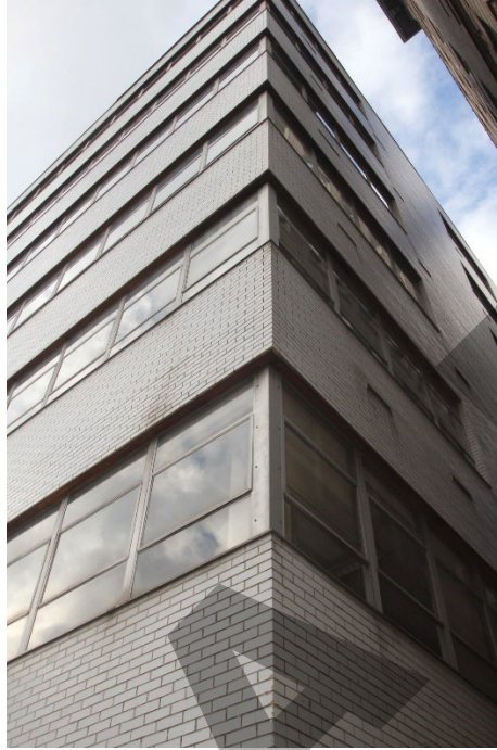
Photo 5 – Northeast corner, looking southwest.
