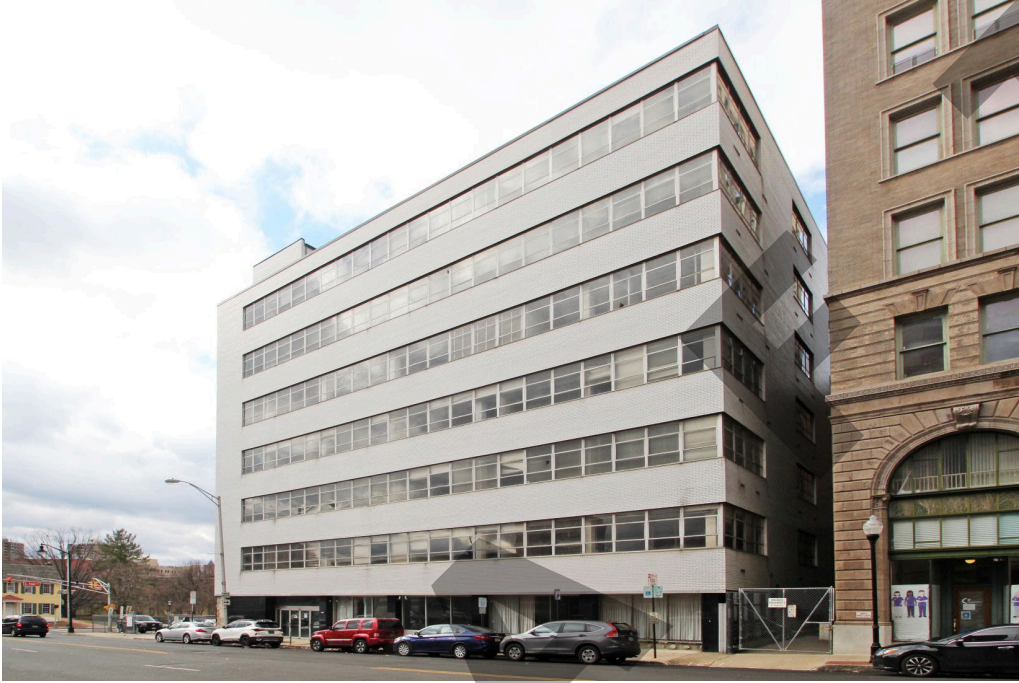
Photo 1 - East elevation, looking southwest.
