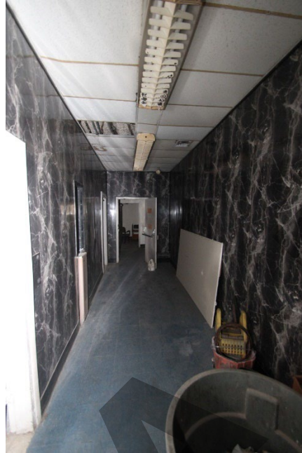
Photo 11 - 1 st floor, hallway, looking west.
