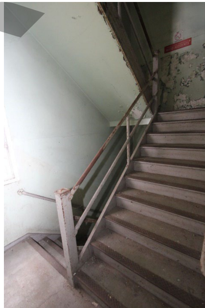
Photo 18 - 2 nd floor, stair, looking northwest.
