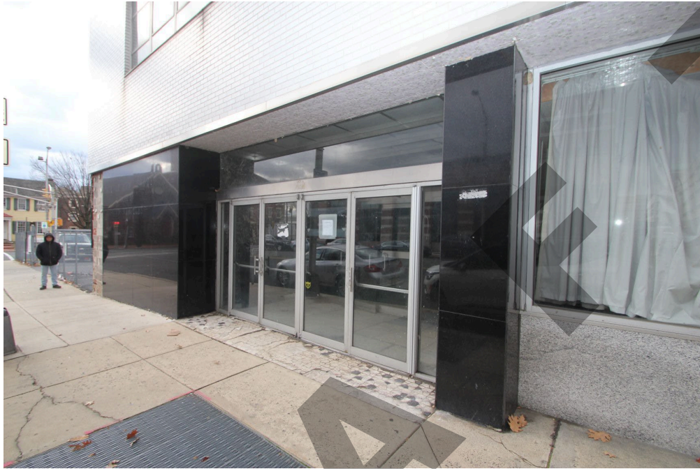
Photo 3 - East elevation, main entrance, looking southwest.
