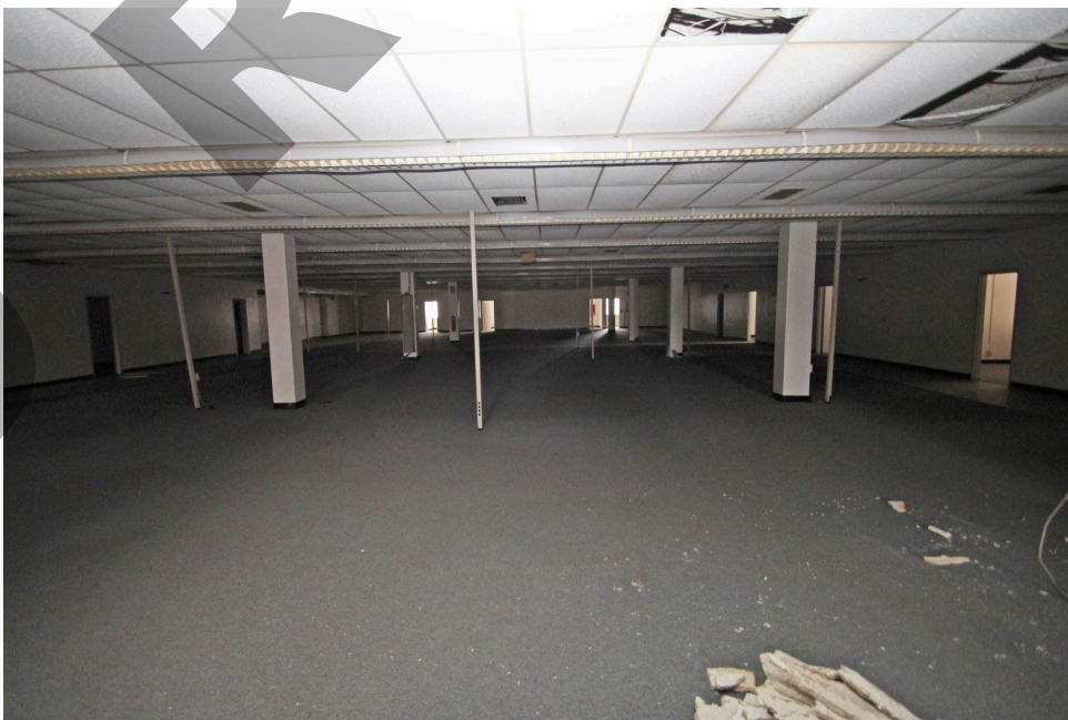
Photo 22 - 6 th floor, office area, looking west.
