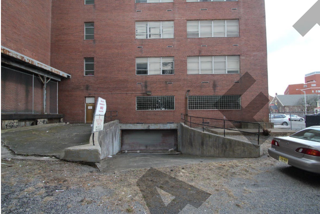
Photo 7 - West elevation, garage entrance, looking east.
