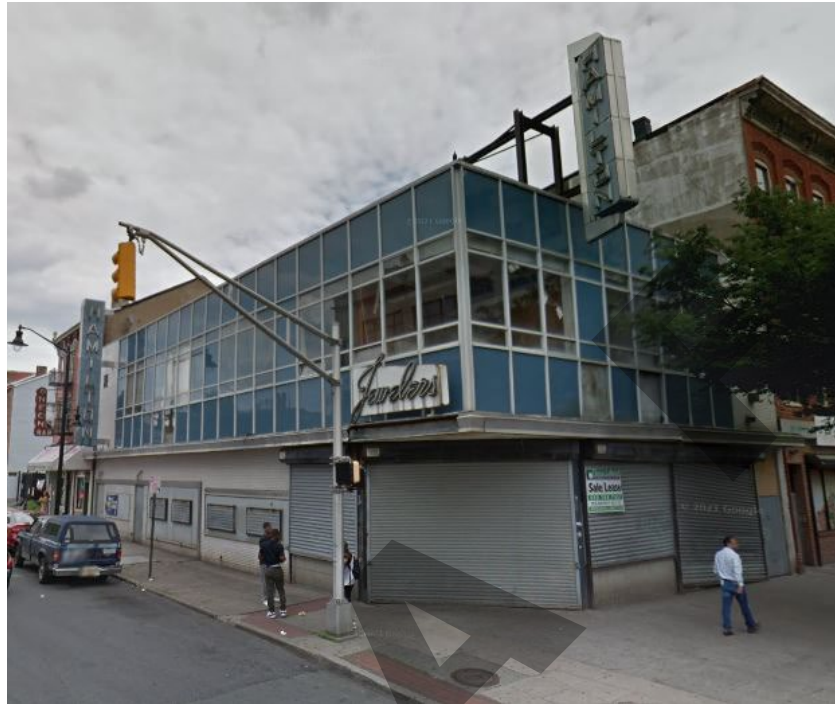
Figure 20 – Hamilton Jewelers Building at the northeast corner of N. Broad and E. Hanover Streets in Trenton, NJ, designed by Louis S. Kaplan and built 1958 (Google Street View).
